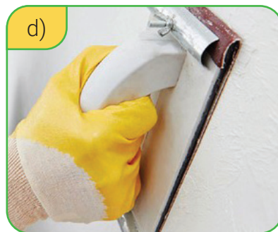
84-rasm. Shpaklyovka surtishning bosqichlari: a) shpaklyovkani mikser bilan tayyorlab olish; b) shpaklyovkani surtish; d) jilvir qog'oz bilan tekislash.
